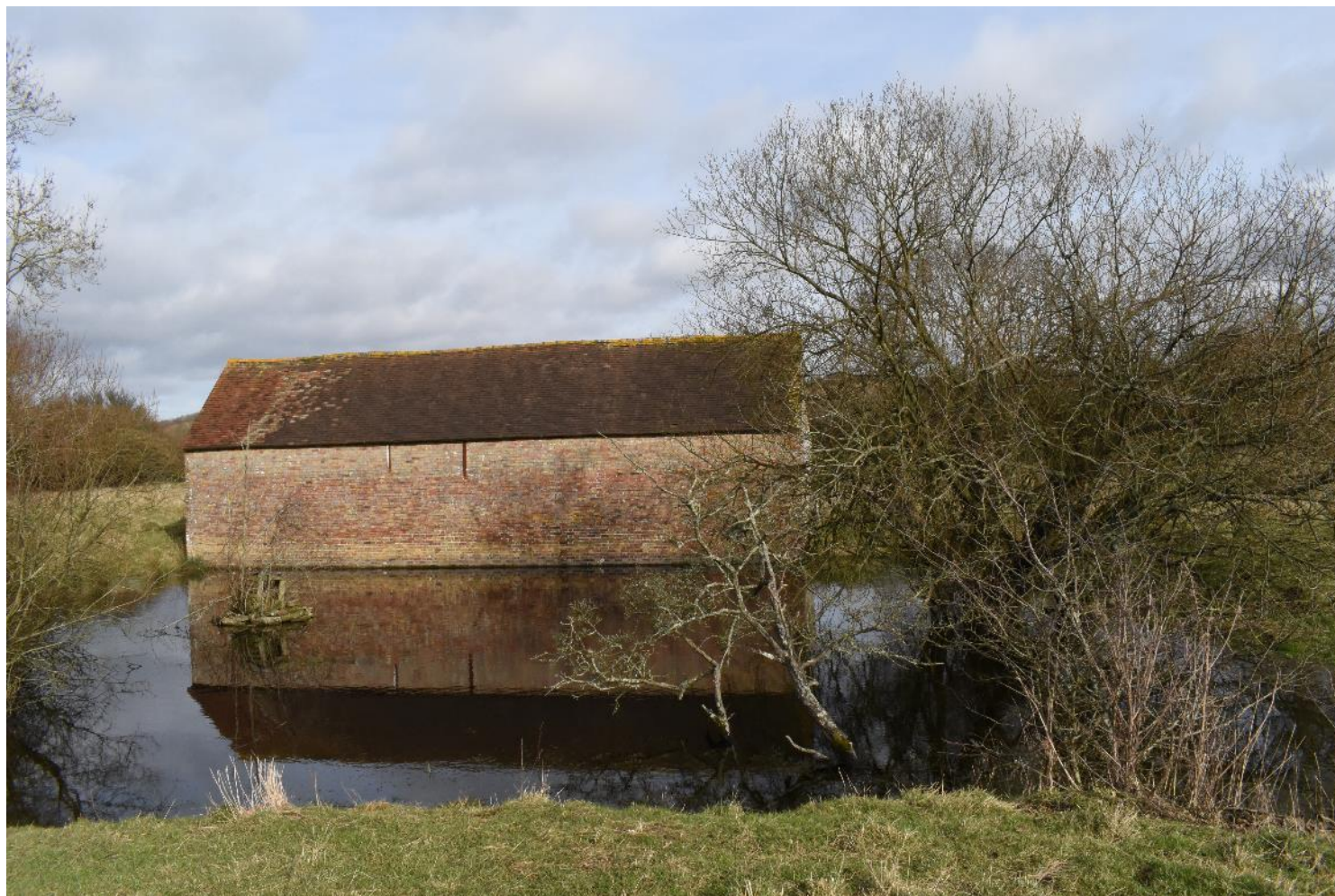
Plate 14: View towards the rear of the cattle shed (facing NE).
