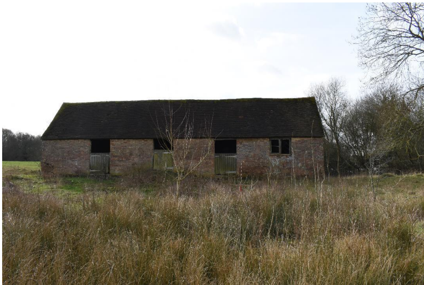
Plate 16: View across the central courtyard area towards the cattle shed, scale 1m (facing SW).
